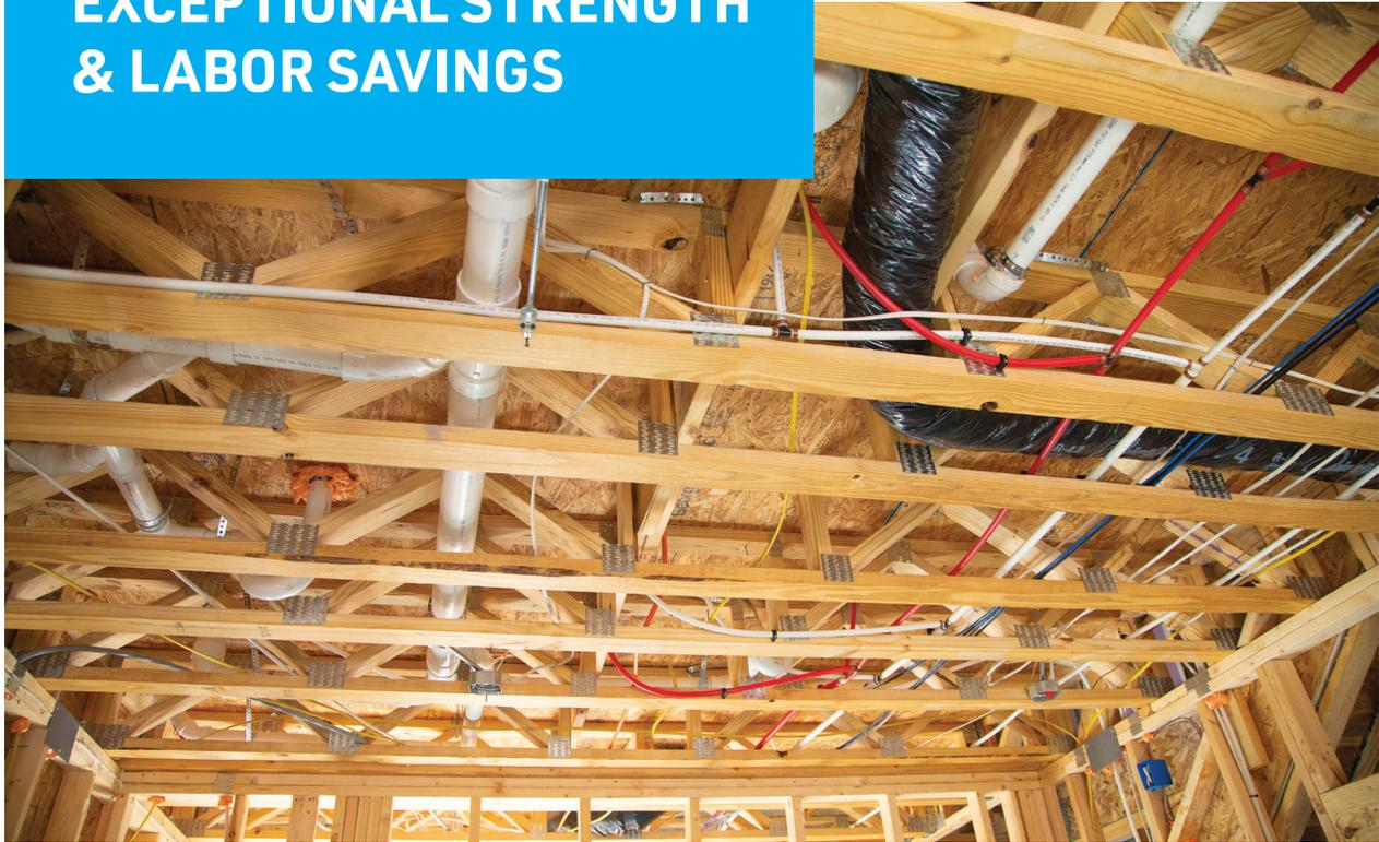
Open web floor trusses deliver faster cycle times, reduced wood materials, and less waste than engineered wood products or dimensional lumber.
