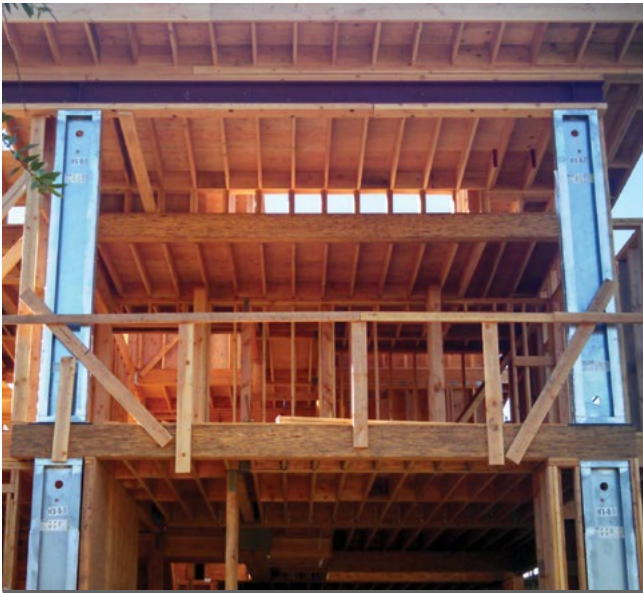
SHEAR WALL PANEL
