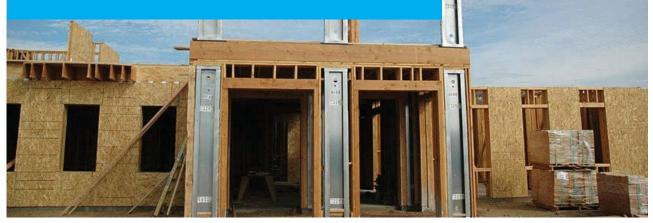
The most cost-effective and narrowest prefabricated shear wall panel in the industry, the MiTek Hardy HFX Shear Panel enables narrower walls and larger openings. The MiTek Hardy "C-Shape" allows trades to insulate and recess fixtures easily.
